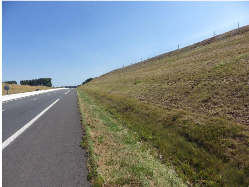
Photo 2 - Cunette enherbée – PR15.42
